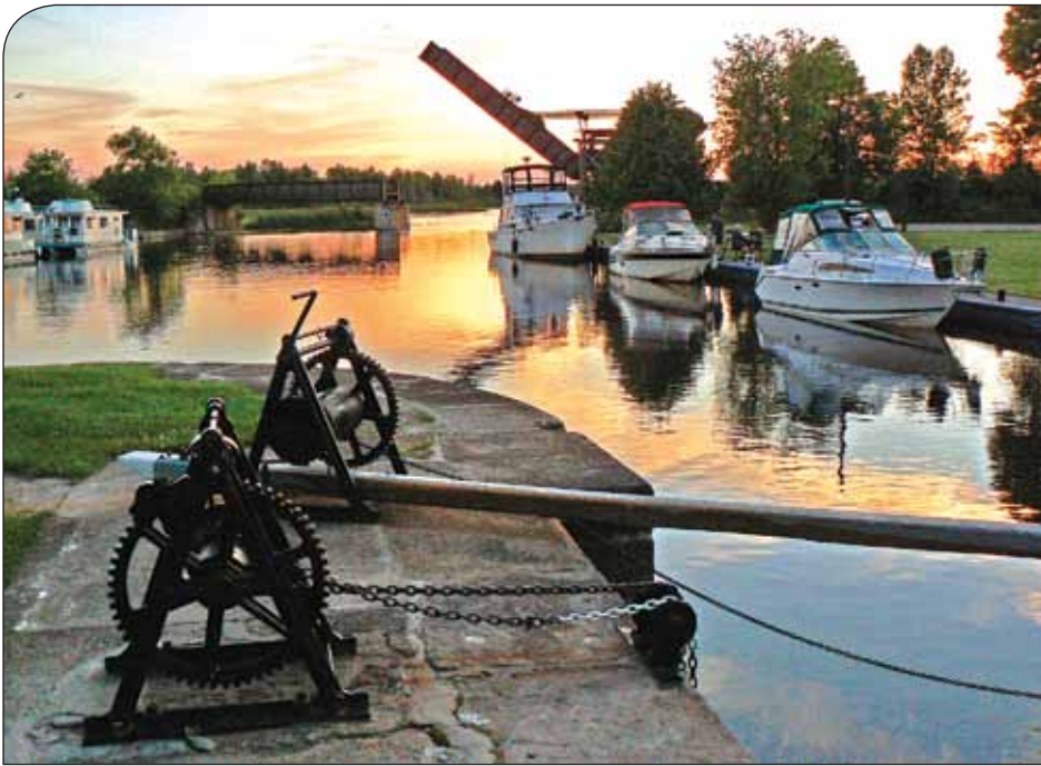
The Smiths Falls Detached Lockstation and Railway Bridge (photo by Simon Lunn)
